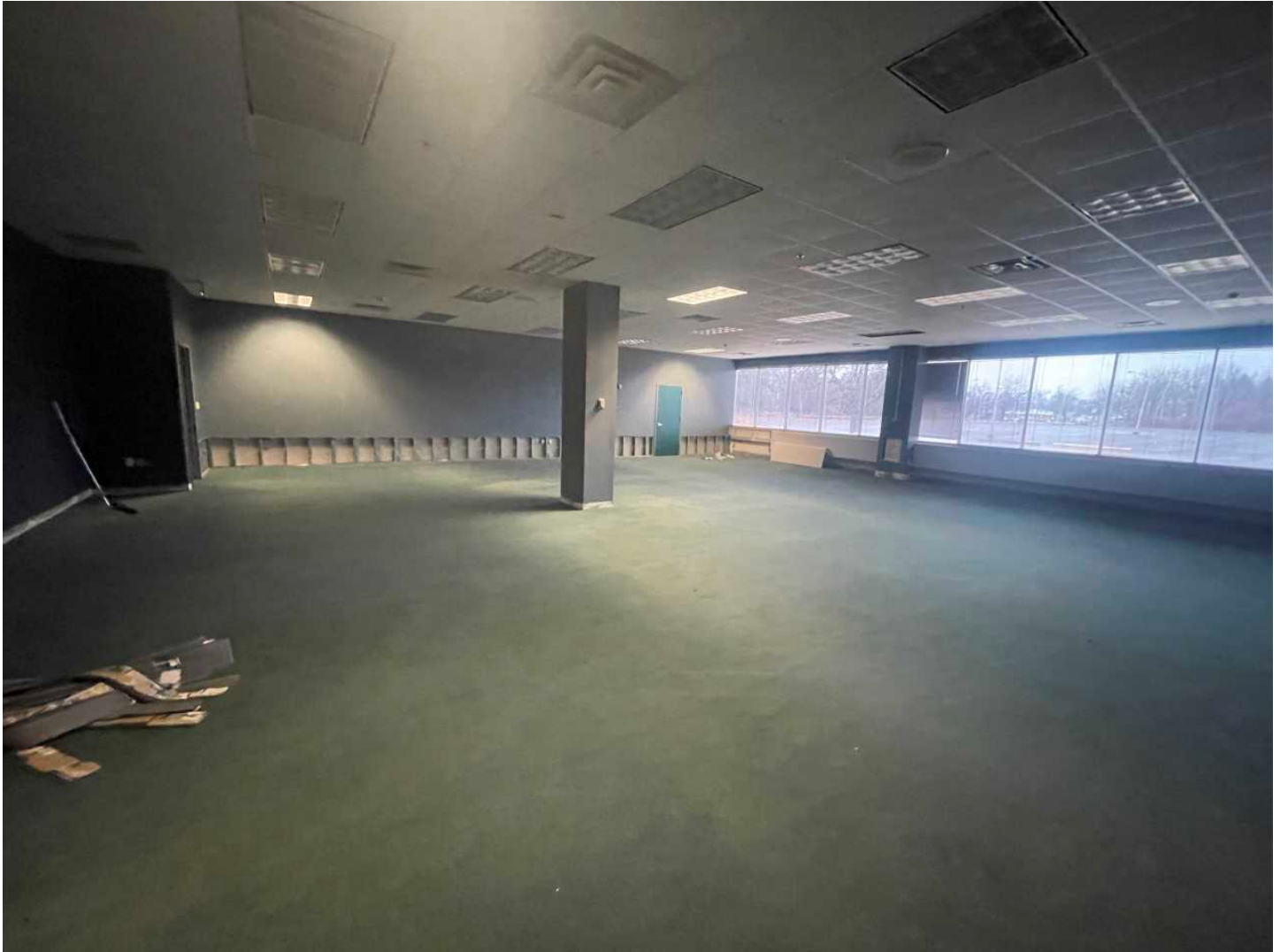
32 33-IMG_9113 Room 2 completed
