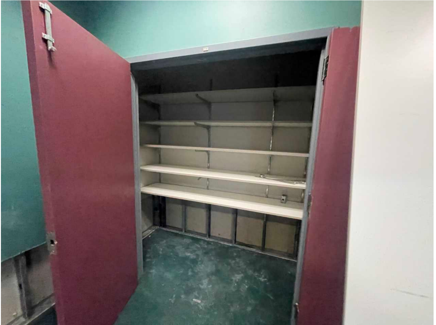
34 35-IMG_9115 Room1 closet completed
