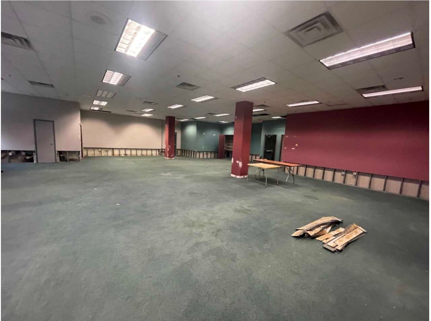
33 34-IMG_9114 Room 1 completed
