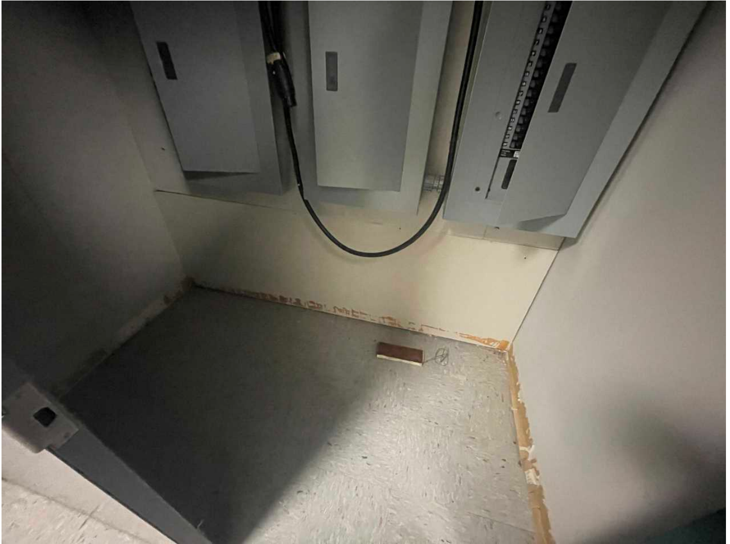
31 32-IMG_9112 Hallway closet completed
