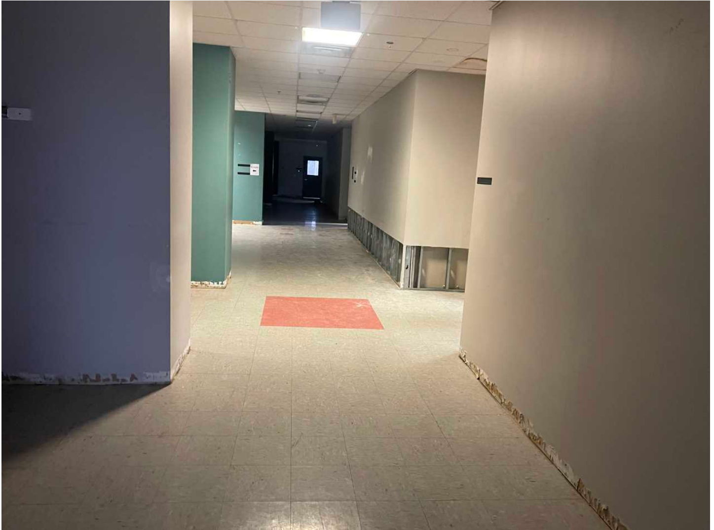
29 30-IMG_9110 Hallway completed
