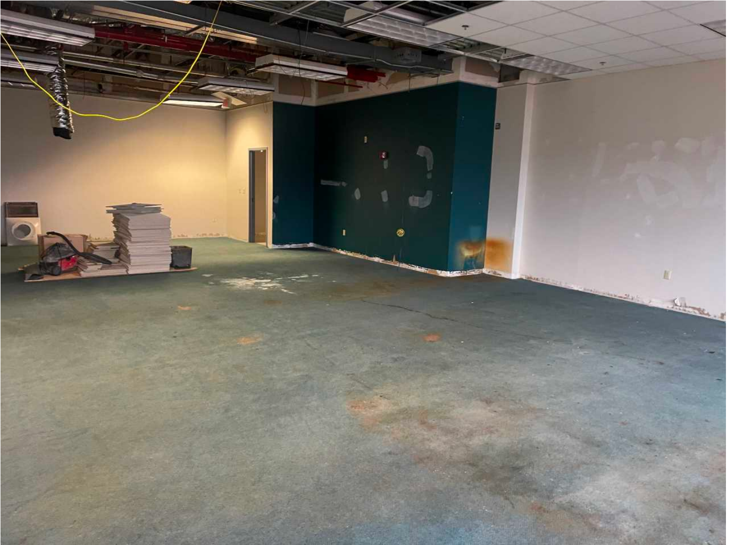
28 29-IMG_9109 Room 4 completed
